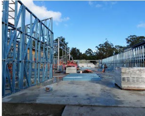
Library – Structural Steel & Lightweight framing
