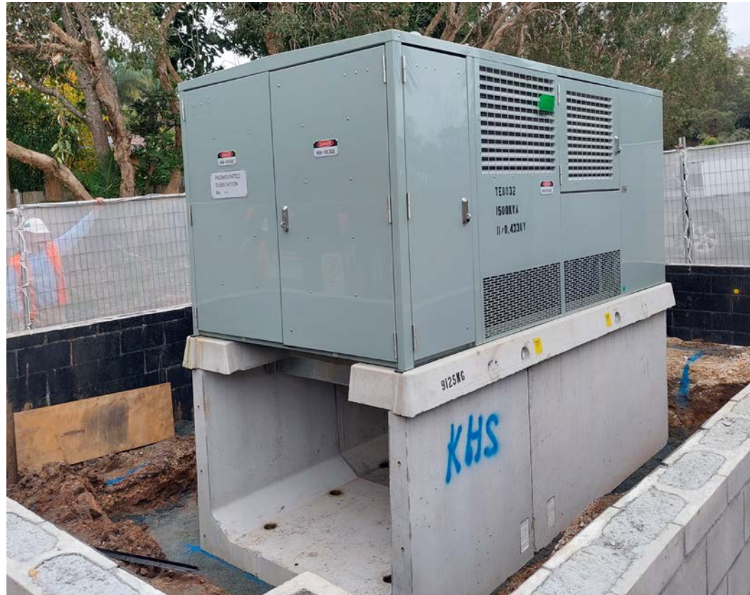
Substation - Culvert and Transformer Installed
