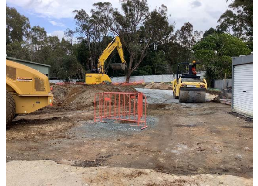
Building O - Pad Cut to Height and Sealed
