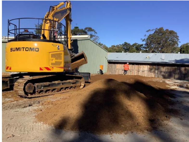
Building O - Earthworks
